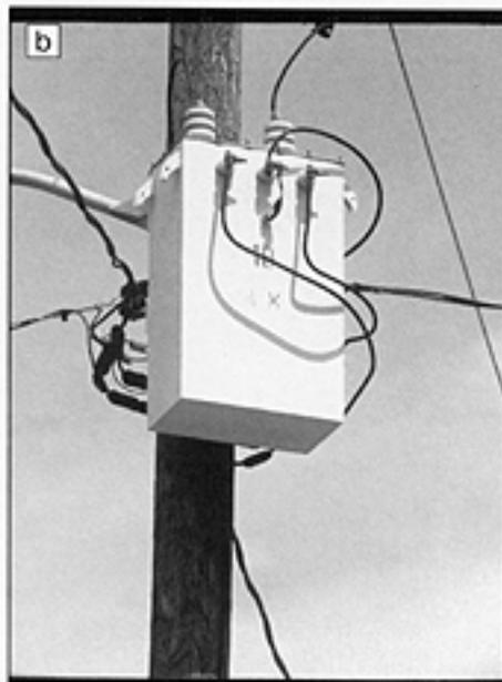
**Figure 1. (a) Experimental General electric pad-mount amorphous -metal transformer. (b) Experimental Westinghouse Electric pole-mounted amorphous metal distribution transformer**
